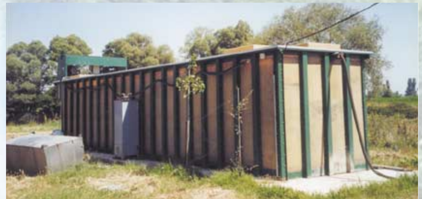
Dairy wastes treatment Plant
